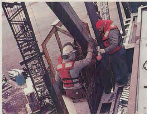
SOF's John Donovan sets charges before blowing bridge. Photo: Courtesy of John Donovan
